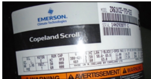
Photo #8 Test unit compressor
