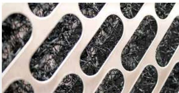
To protect the condensers all MECOCHILL chillers include progressive composite fiber mesh filters which can be easily removed for service and cleaning. Filter could be removed from its own housing outside the canopy to be washed with water or cleaning fluids.
